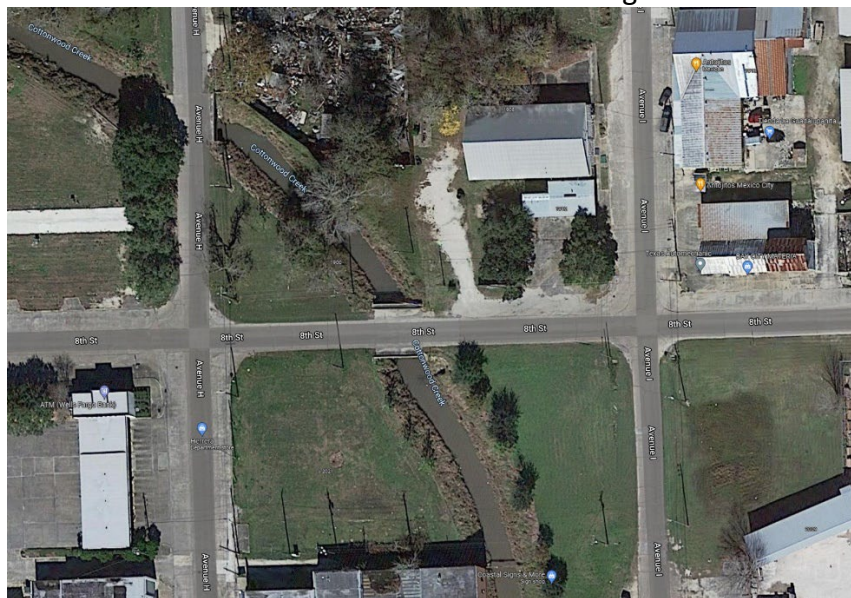
8 th St & Cottonwood Creek Bridge
