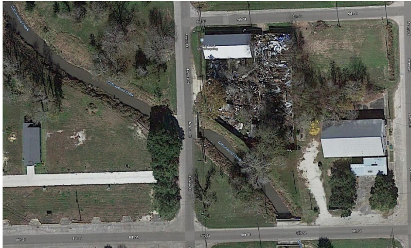
Ave H & Cottonwood Creek Bridge 1
